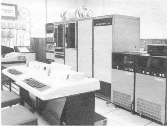
A view of the HP-3000 Series II model 8 used in ESL's IDIMS facility.
